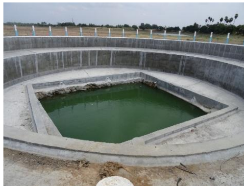
Figure 29 Sub surface groundwater recharge
